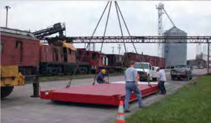
Module A is unloaded from the truck and placed on the foundation. Module B is then unloaded and fitted with Module A.
